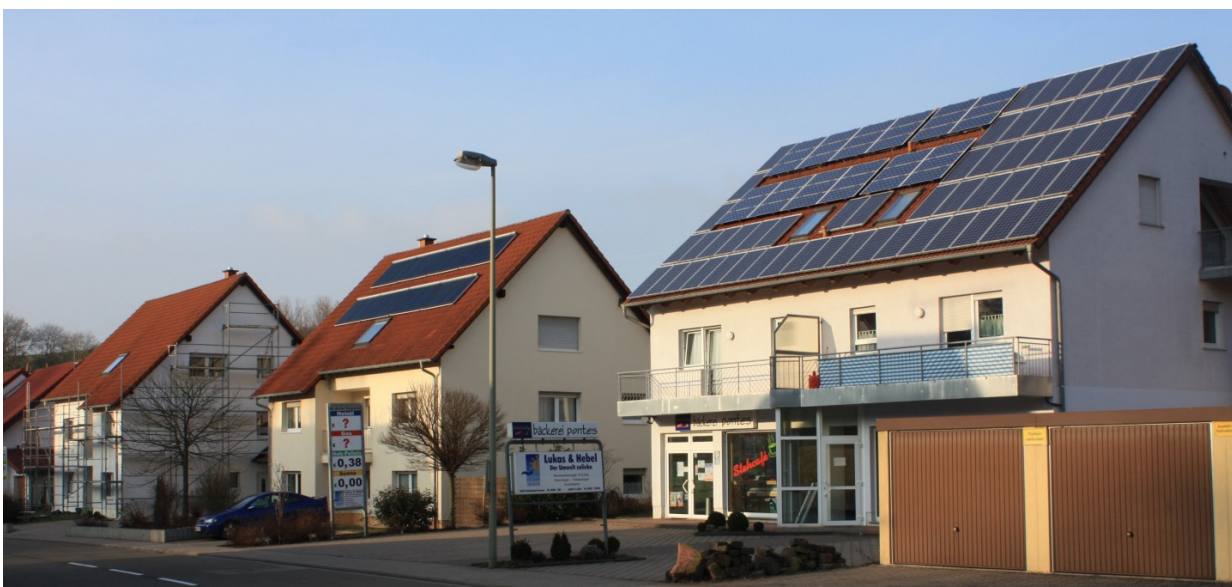
Figure 2: Building site in Reichenbach-Steegen
